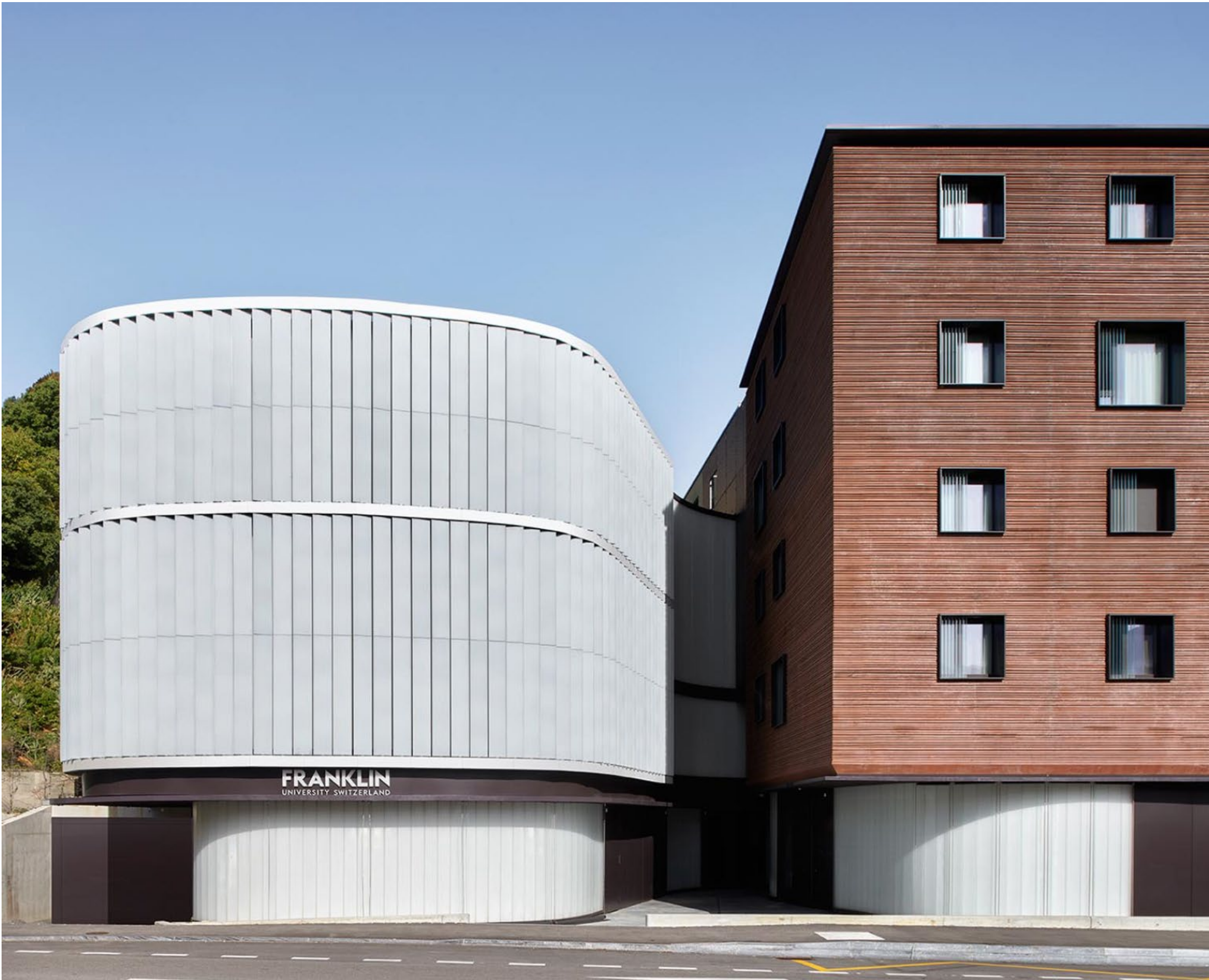
Fig. 1: Franklin University Switzerland dynamic solar shading system, Sorengo. Credits: Flaviano Capriotti Architeti.
